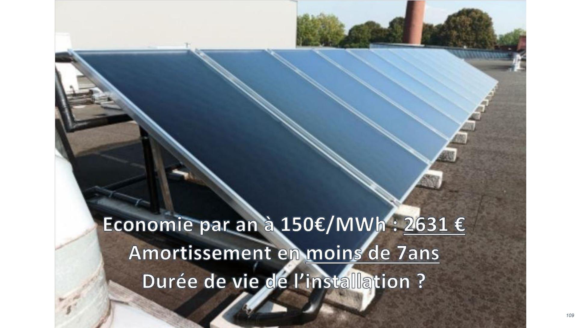
A photograph showing a row of solar collectors (likely flat-plate collectors) installed on a rooftop. The collectors are blue and mounted on a metal frame. The background shows a building and some trees under a clear sky.
